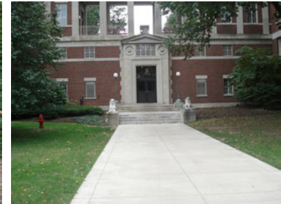
F: Tunnel Entrance
